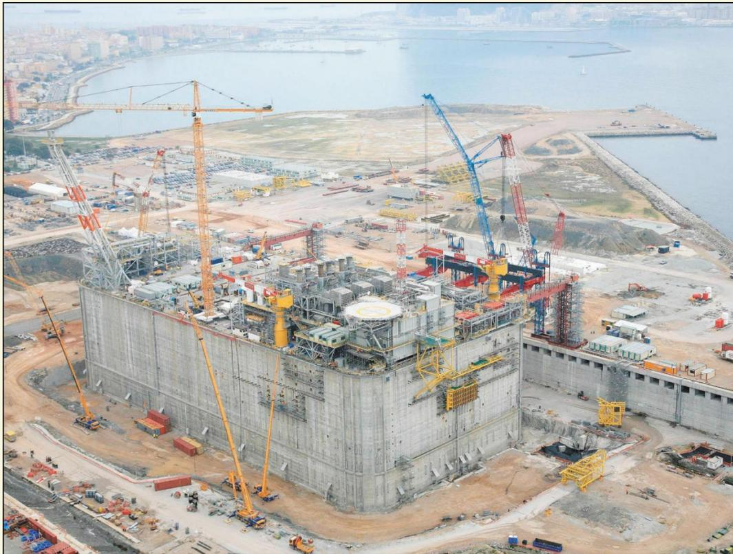
A FLOATING concrete platform housing an offshore regasification plant will be floated out of the port of Algeciras this summer and towed to the Adriatic Sea, where it will operate anchored off the Italian coast.
